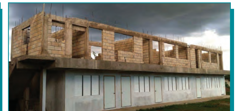
School construction, to date
